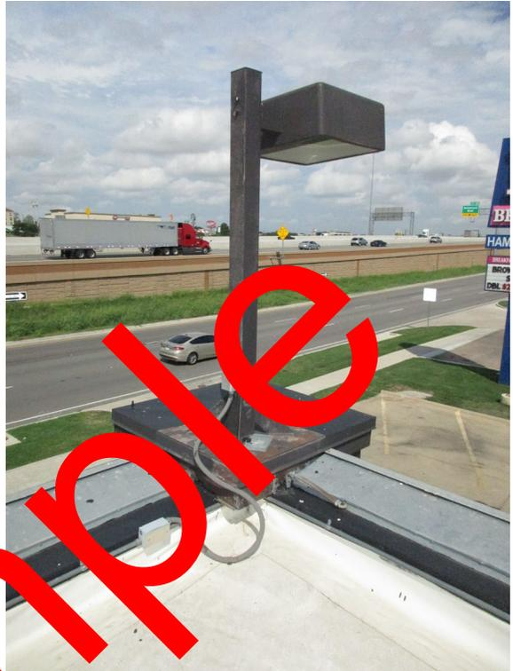
**PHOTO #13** – Typical view of parapet mounted light fixtures.
