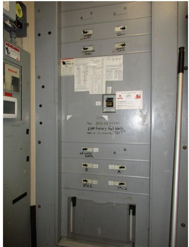
**PHOTO #20** – View of main electrical panel and breakers.
