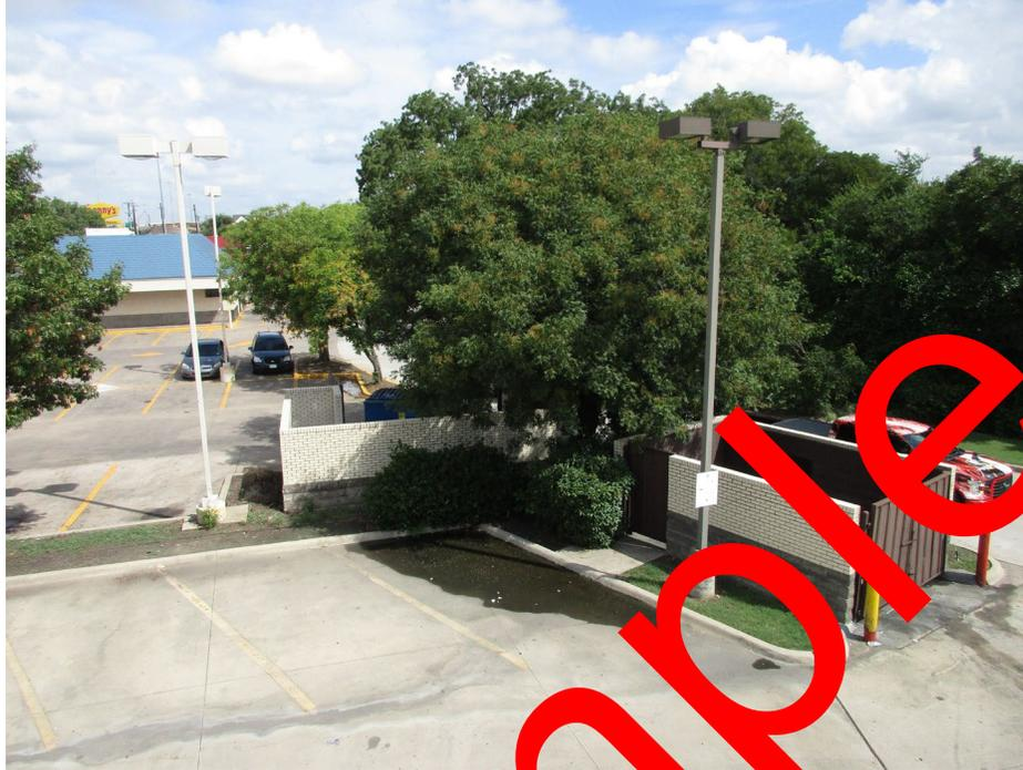
**PHOTO #5** – View of dumpster enclosure and pooling water in north parking lot.
